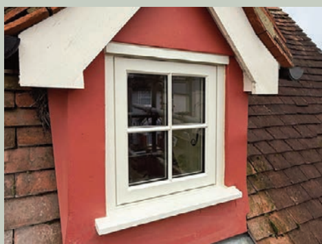
Lipped casement windows with bar detail.
