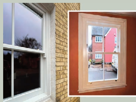
Box sash – internal view includes brass fittings.
