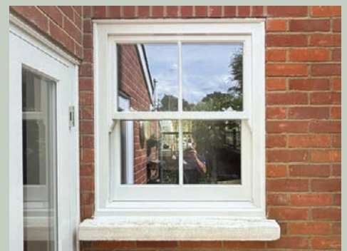
Spring sash – installation on existing stone cill.
