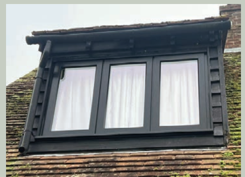
Large three-sash flush casement dormer window.
