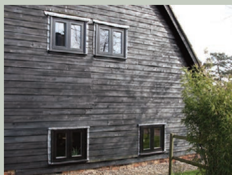
Flush casement windows with lead flashing.
