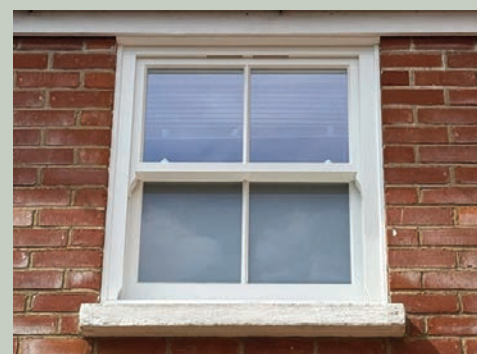
Spring sash – design includes frosted privacy glass.
