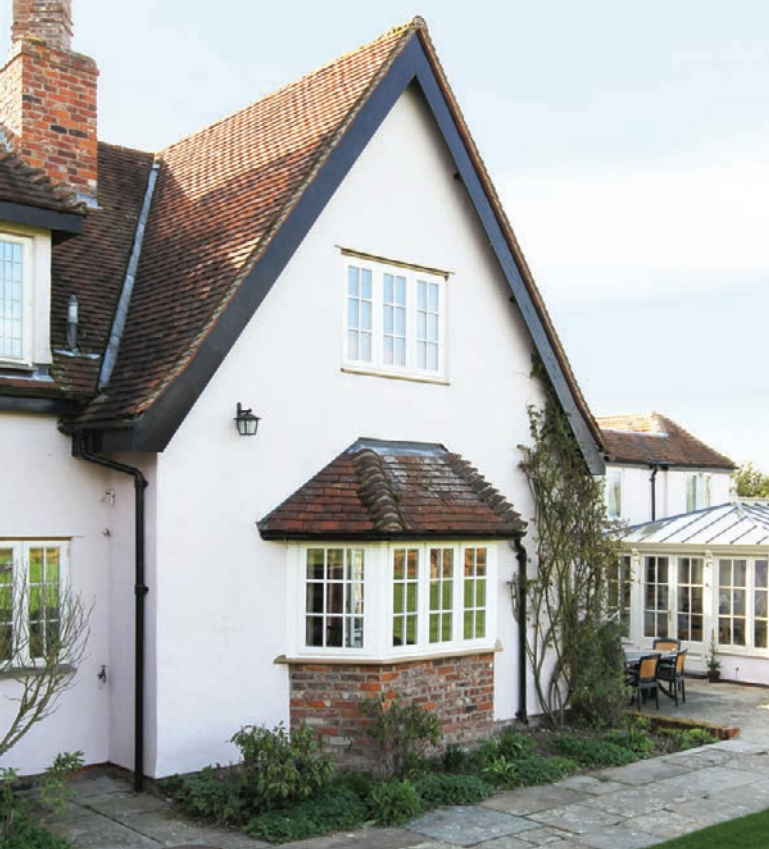
Lipped casement bay window with Georgian bar in white produced to match the existing windows in this country home.
