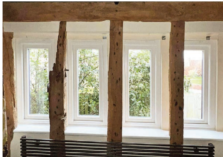
External and internal (below) photographs show the installation of flush casement windows between the beams of this barn conversion.
