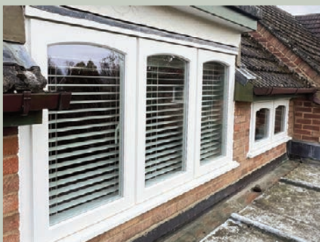
Timber lipped casement with arched detail.
