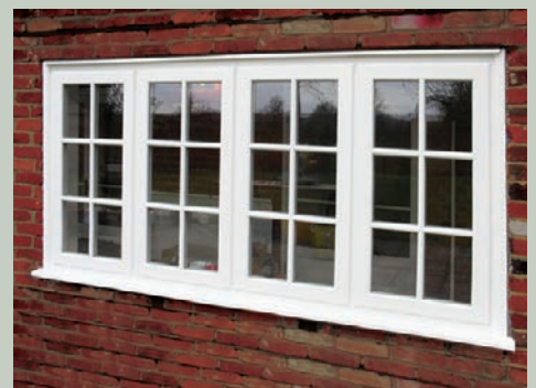
Two opening sashes and two central dummy sashes.
