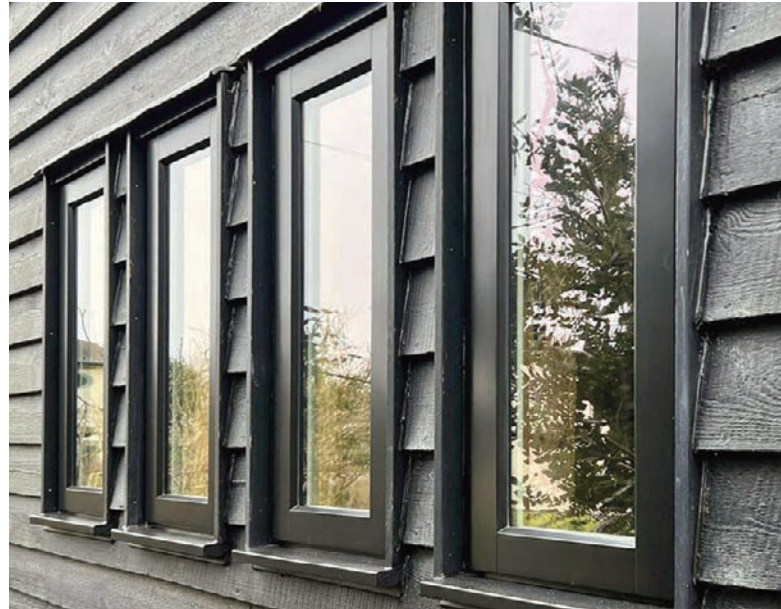
External and internal (below) photographs show the installation of flush casement windows between the beams of this barn conversion.
