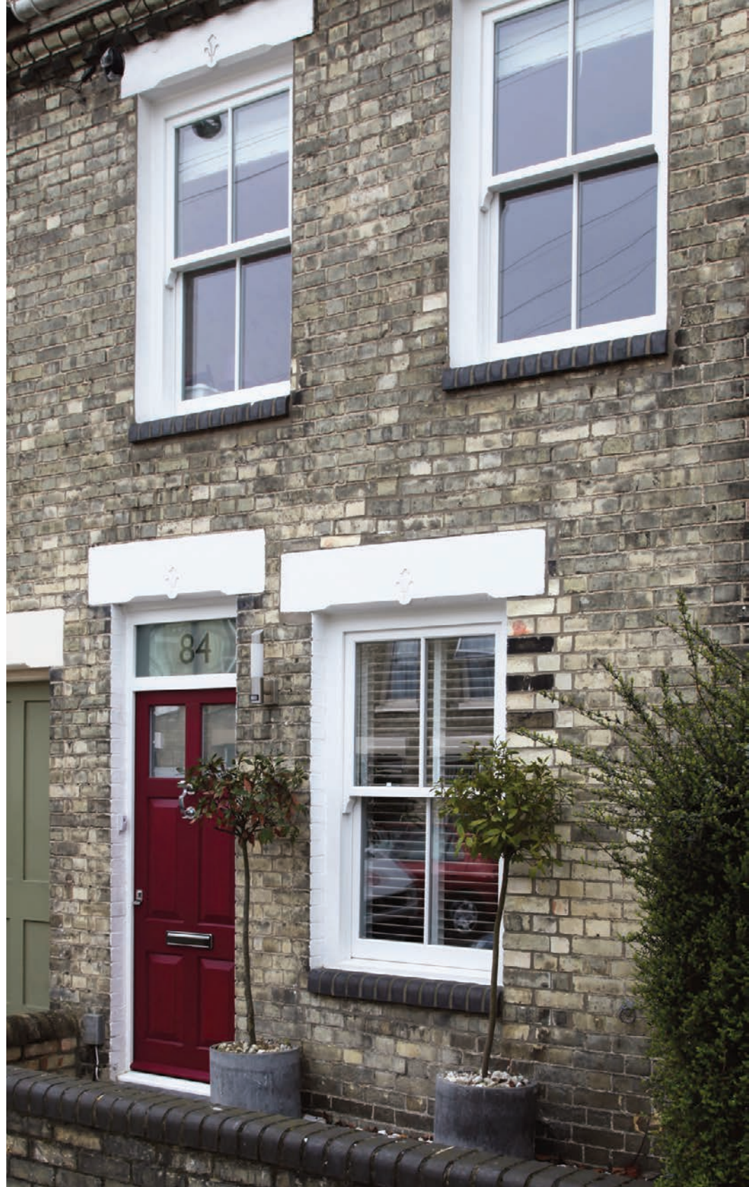
Box sash – picture perfect box sash replacement project carried out on this stylish city centre terraced home.
