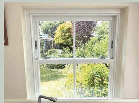
Spring sash – picture shows restrictors in top sash.
