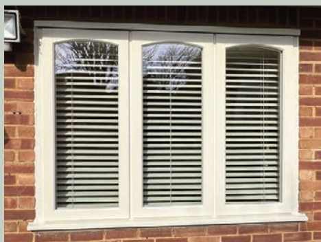
Lipped casement window with arched sash detail.
