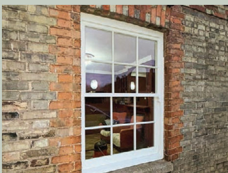
Box sash – classic six over six glass pane design.
