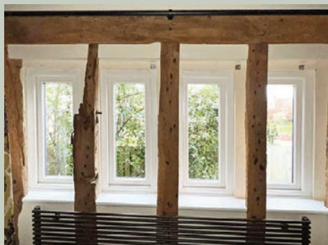
Flush casement sympathetically installed into barn.
