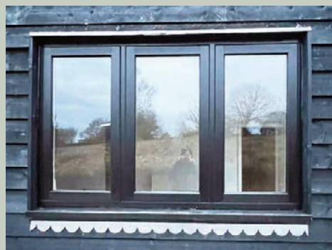
Window featuring scalloped lead work to cill.
