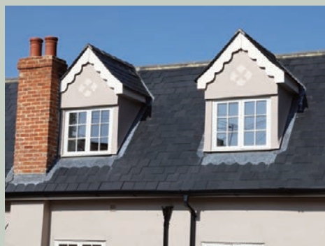
Lipped casement windows with Georgian bar.
