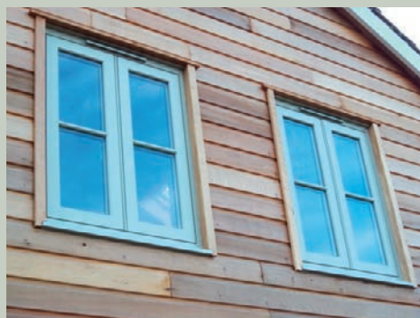
Flush casement with mid-rail to create cottage style.
