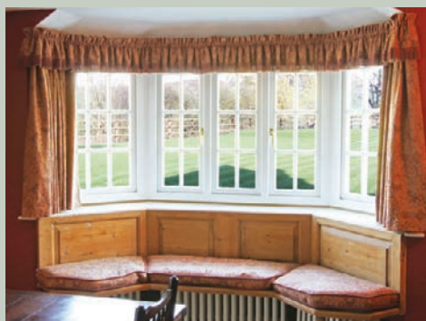
Three section 135° lipped casement bay window.
